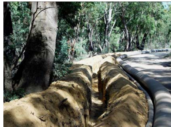
Pipeline being laid between Springvale Colliery and Wallerawang Power Station.
