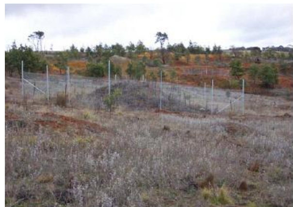
Secured shafts at Blayney Copper Mine
