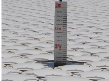
Water level monitoring
