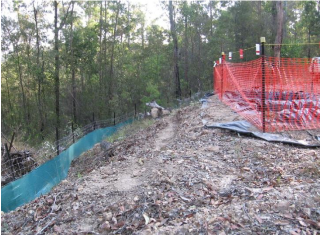
Sediment fence on down slope side of plastic-lined sumps
