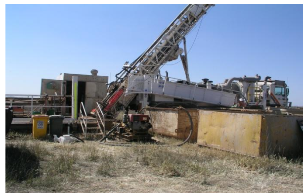
Rig with barge tanks
