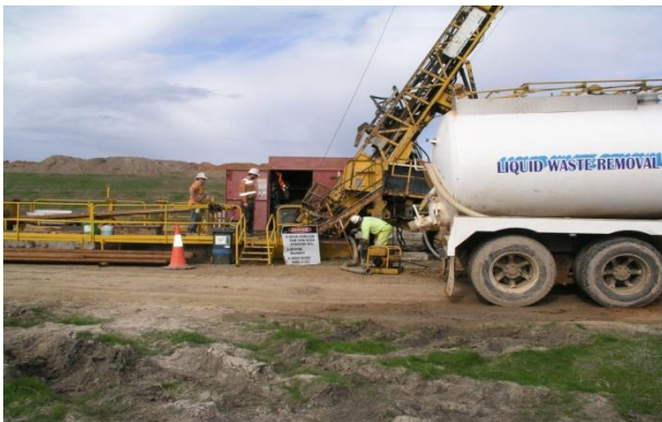
Vacuum truck pumping out barges and collar trough
