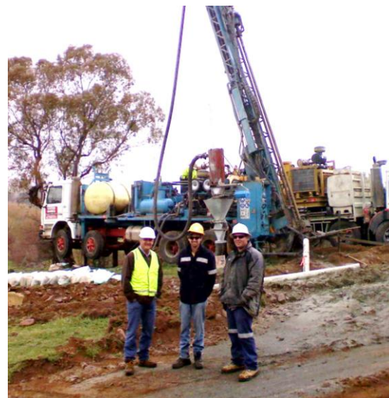
RC drill rig on steep, high rainfall terrain
