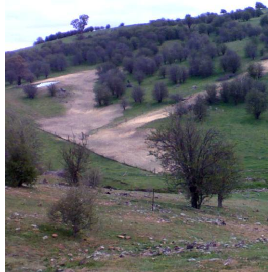
Steep terrain exploration-disturbed areas seeded and straw mulched
