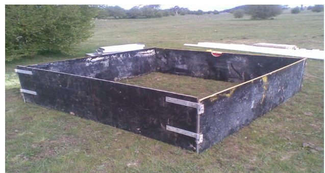
Form-ply sump showing hinges
