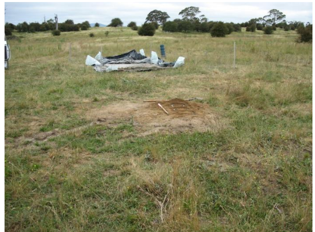
Drill site on completion of hole showing minimal impact and sump liner drying out
